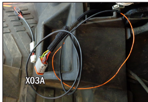
Fig. 36: X03A terminal re-assigned and harness routed into the cabin
